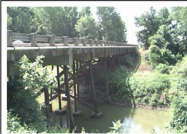
Bridge crossing Big Bayou Meto
