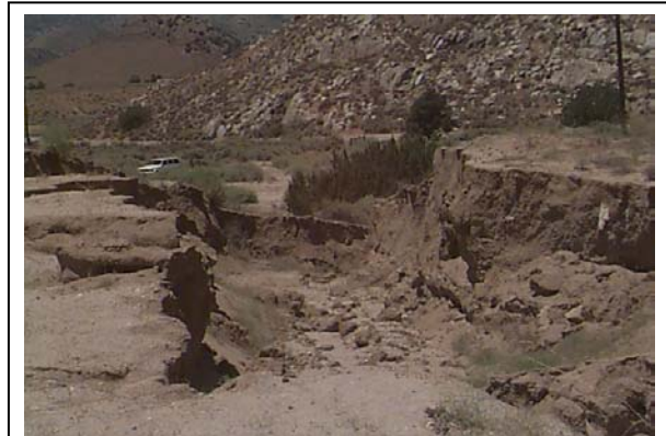
Severe headcut on Cyrus Canyon
